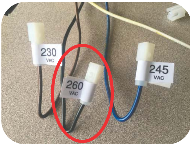
New tap to handle the higher voltage peaks.
